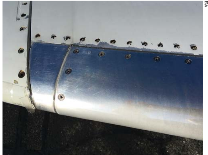
The wing sealant along this CRJ’s leading edge shows clear signs of deterioration and protrusion into the boundary layer. The aircraft’s Configuration Deviation List contains a “weight penalty” to be applied to takeoff due to the lessened lift created by the negative effect on the wing’s boundary layer.
