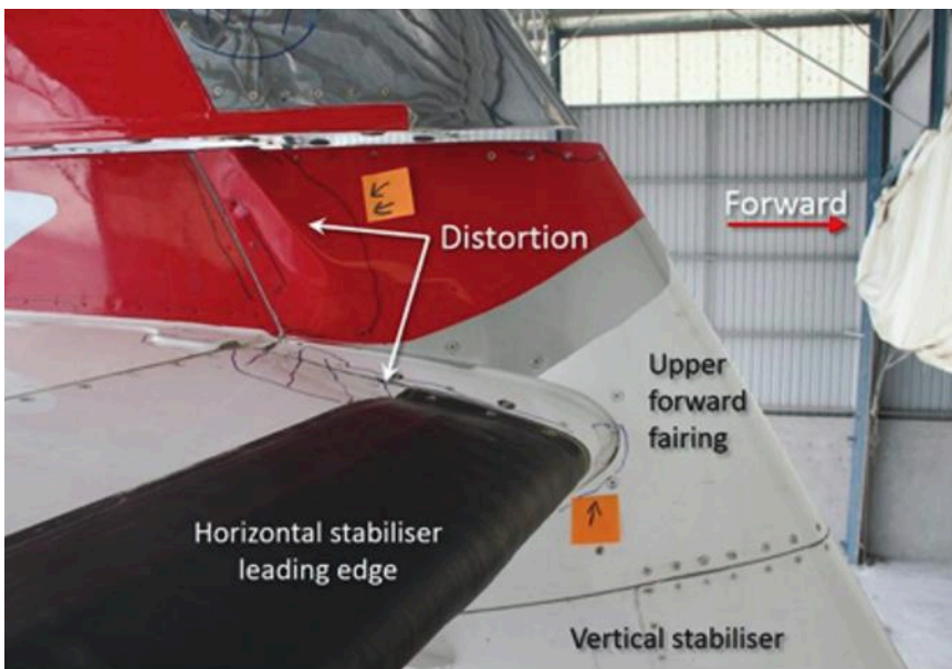
Upper tail plane of VH-FVR showing damage to horizontal and vertical stabilizers that was evident when the damage was identified five days and 13 flights after the inflight upset/pitch disconnect and associated maintenance.
